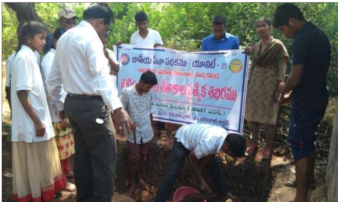
The NSS III Unit (commerce) participating in construction of Water Harvesting Pits on 30-01-2017 at Marripally Gudem Village
